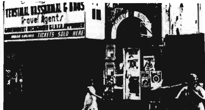
Remains of the burnt out Kishore building at 523 Kalbadevi Road.
