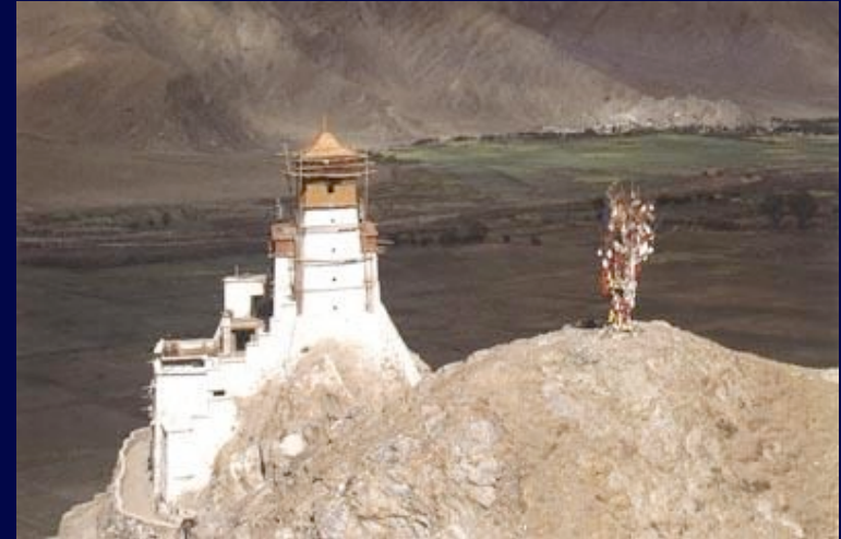
Good structure from west shot
